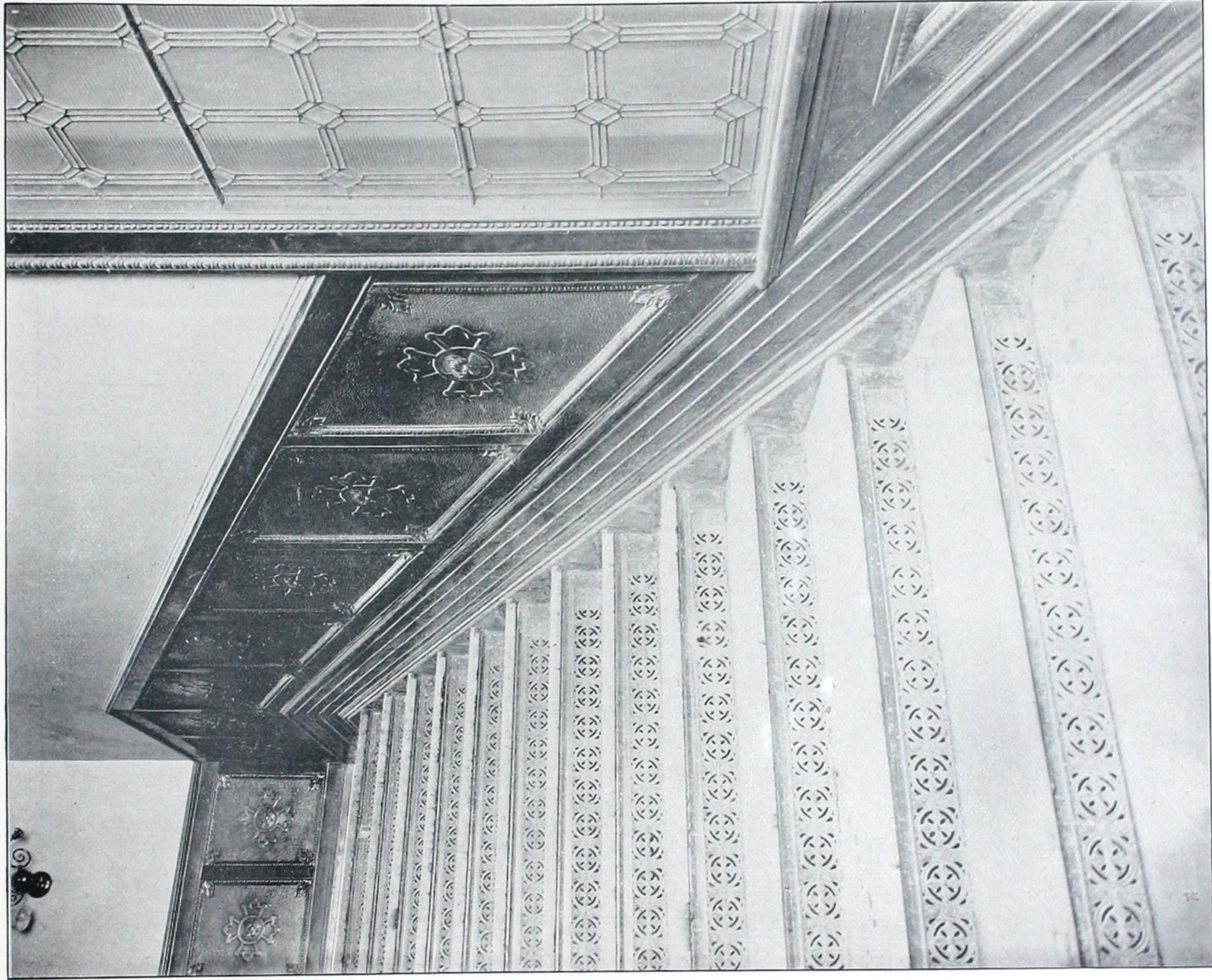
Fig. 148.—Interior View, Temple Building, Toronto.
